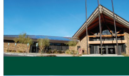
SolarGenerations installation at Boy Scouts of America, Las Vegas
