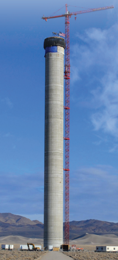
Crescent Dunes Solar Under construction near Tonopah, Nev.
