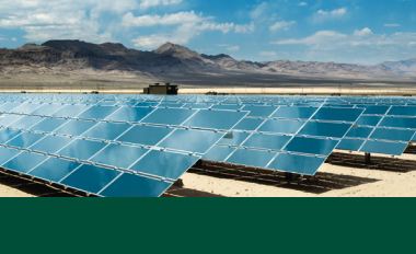
Silver State Solar North near Primm, Nev.
